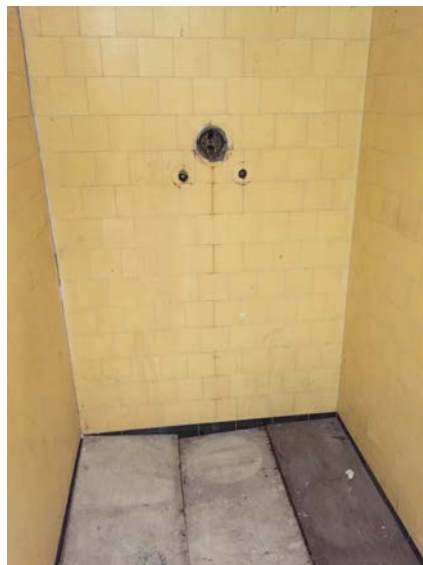
Pre-abatement (men's restroom)
