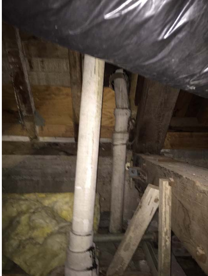
Asbestos-cement pipes, attic.
