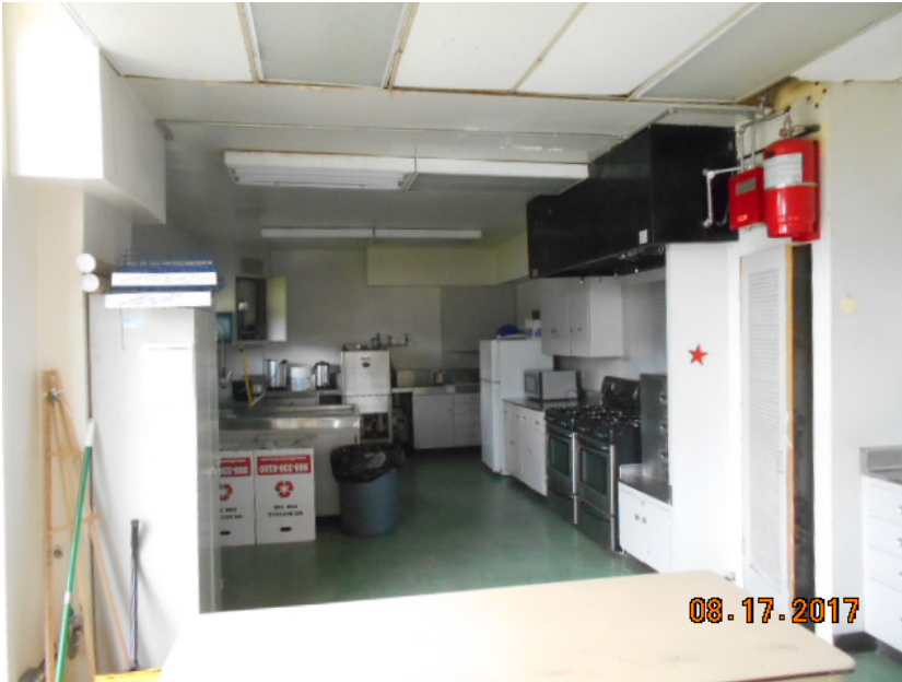
12” flooring and mastic, kitchen
