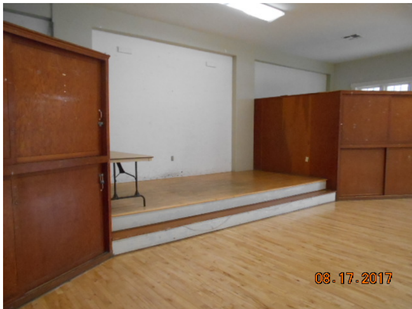
Concealed felt paper under auditorium floor – assumed positive.
