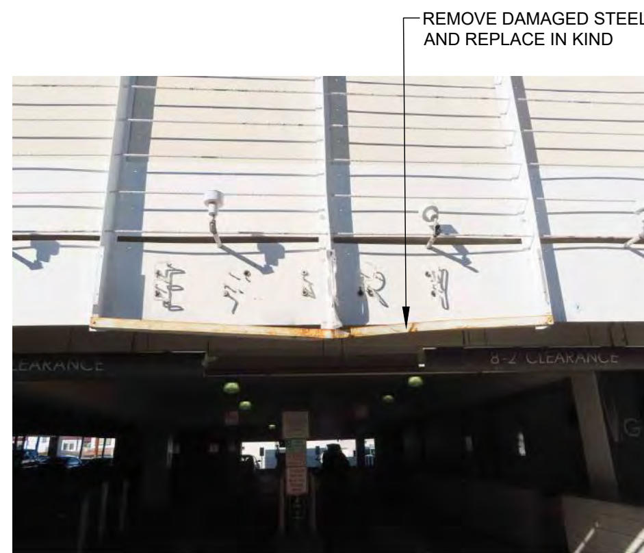
43.7 SOUTH ENTRANCE IMPACT DAMAGE
