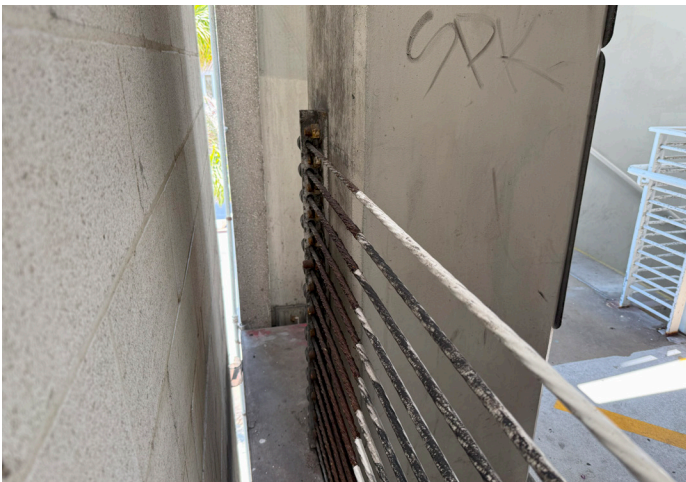
Detail 43.4 REPAIR EXISTING BARRIER CABLE
