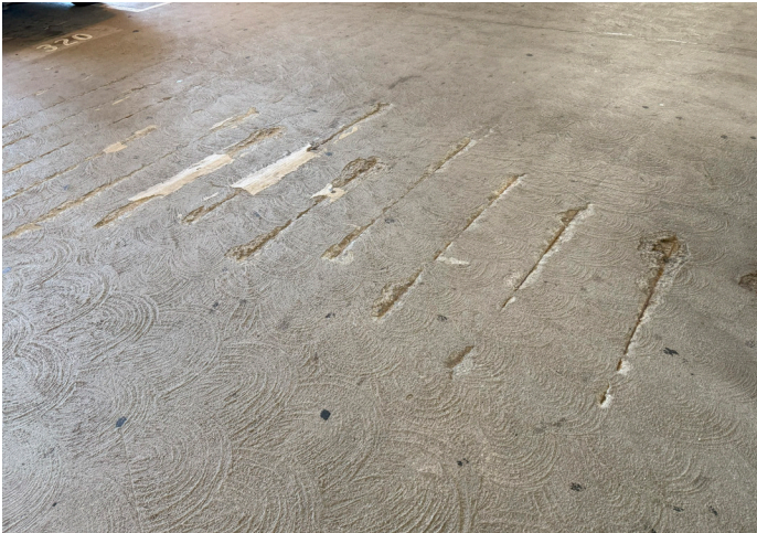
Detail 3.1 FLOOR REPAIR – PARTIAL DEPTH
