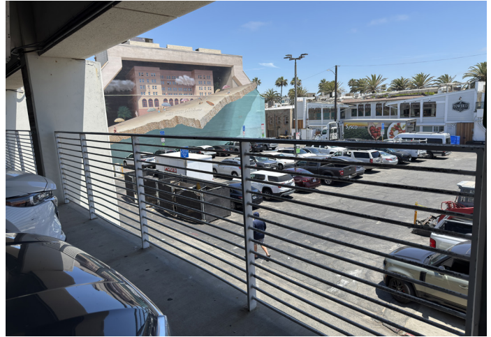
Detail 40.6 REMOVE EXISTING GUARD RAIL (SECOND FLOOR - SOUTH ELEVATION)
