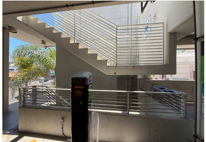
Detail 43.2 REMOVE, SALVAGE AND INSTALL EXISTING GUARD RAIL
