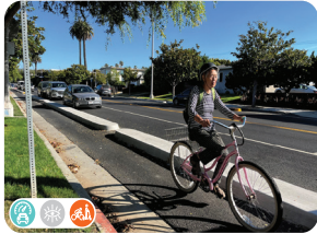
Separated Bike Lanes with Concrete Buffers Creates comfortable, connected networks to make bicycling more attractive and accessible to people of all ages and abilities.
