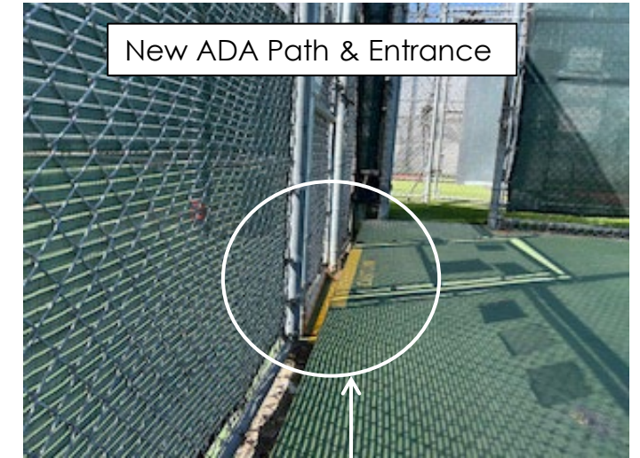
Existing Dropoff between Basketball & Pickleball Courts
