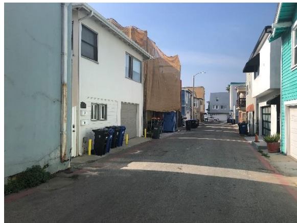
Figure 19: Typical residential buildings along 10 th Court, view west.
