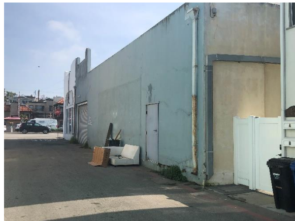
Figure 11: North façade, view southeast.
