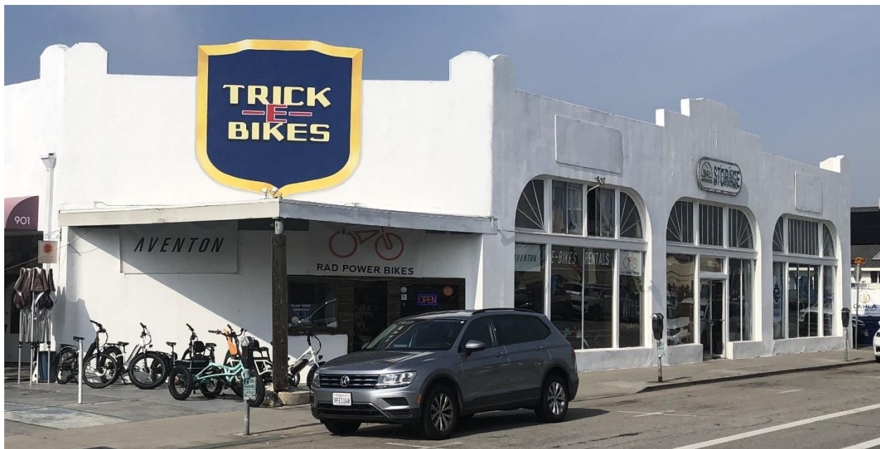
Figure 5: Primary façade (right) and southeast angled corner façade (left), view northwest.
