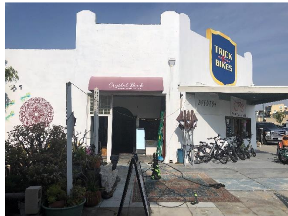
Figure 14: South façade, east end, view north.
