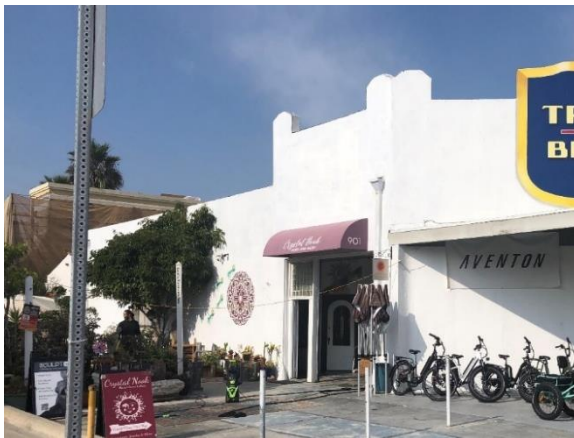
Figure 13: South façade, view northwest.
