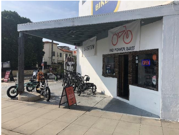
Figure 6: Southwest corner, view west.
