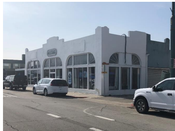
Figure 9: East façade, view southwest
