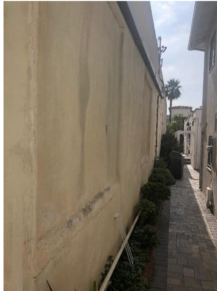
Figure 12: Rear (west) elevation, view south.
