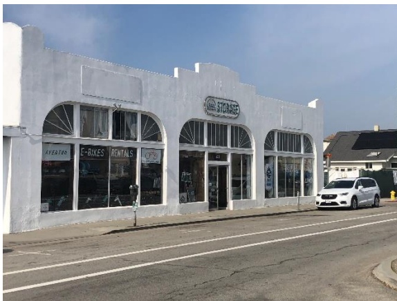
Figure 8: East façade, view northwest
