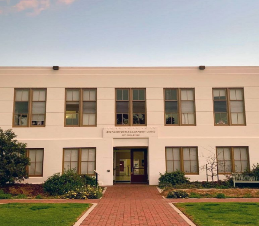
CIP 630: Community Center Gasline Repairs
