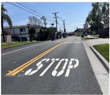
This project provides traffic striping and pavement marking improvements and modifications to improve safety and visibility. This project will help address thermoplastic striping needed which the City is not capable of installing directly.
