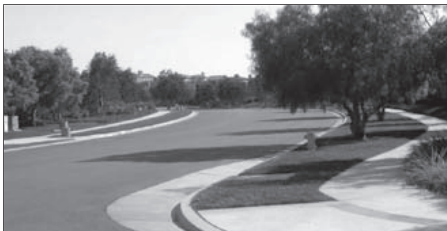
Figure 4. Chambord Road before restriping.
