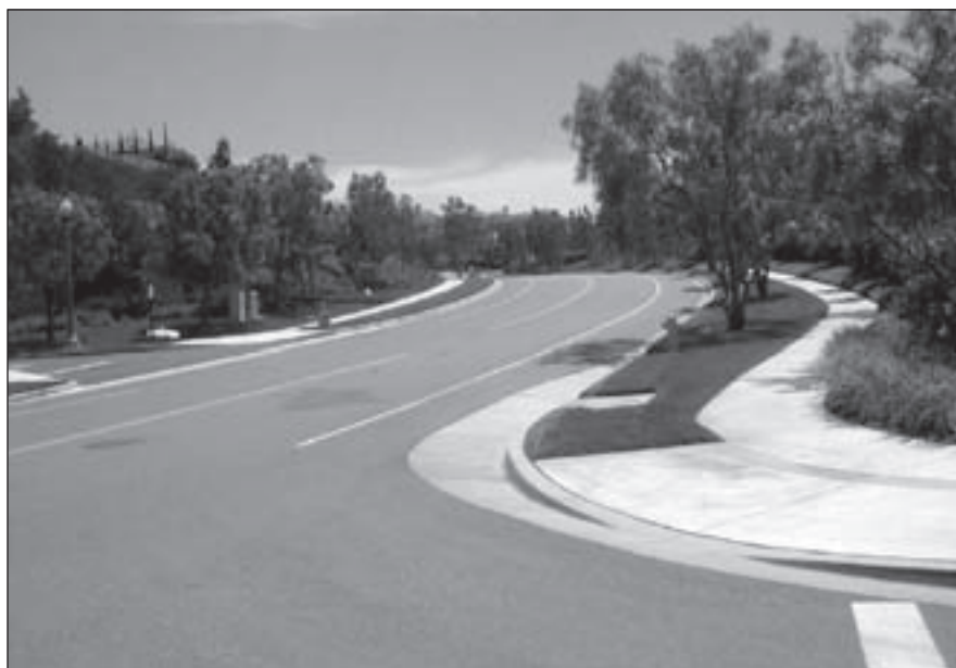
Figure 1. Typical traffic calming striping.
