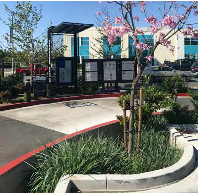
Storm water runoff is collected in planters.
