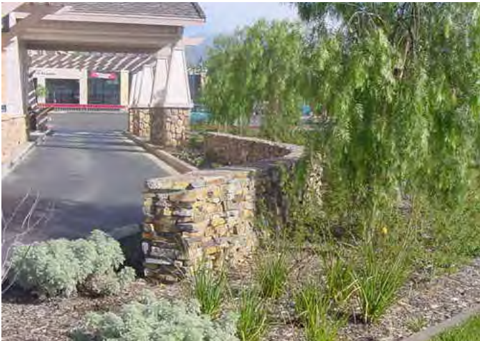
Decorative wall and landscaping provides buffer and screens stacking lanes.
