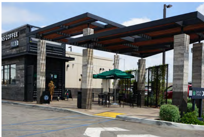
Covered walkway adjacent to building utilizes complementary materials of the building.
